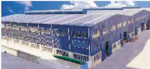
Monforts Fong's new plant
